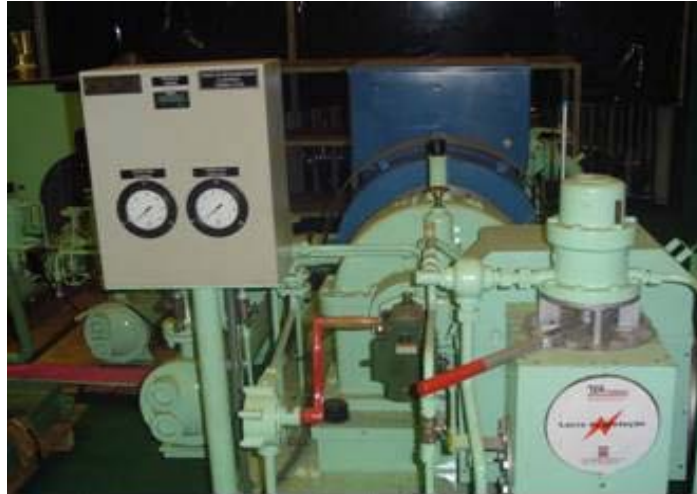
Figure 2 – Turbo-generator produced for TGM and WEG Companies (CENBIO, 2006)
